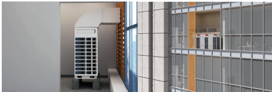
Installation of duct
